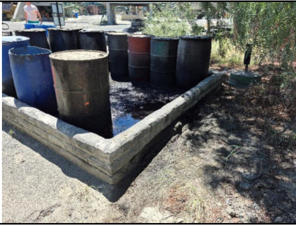
Hazardous waste storage area where bund wall integrity needs constant management
