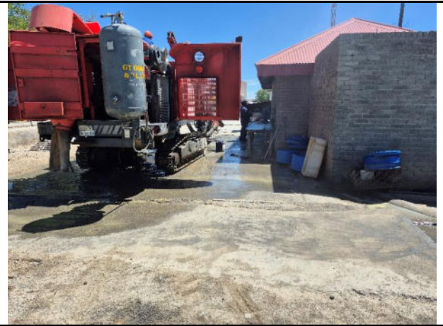
Washbay runoff to be directed to the oil sump
