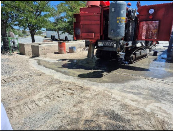
Washbay runoff to be directed to the oil sump
